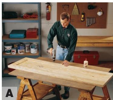
**A** Attach the long and short blocking pieces to the bottom panel, flush around the perimeter, with glue and 1-1/4-in. flathead wood screws. Drill pilot holes for the screws first.
