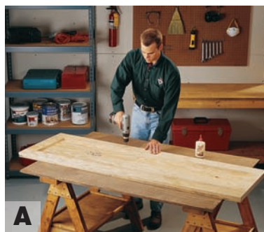
A Attach the long and short blocking pieces to the bottom panel, flush around the perimeter, with glue and 1-1/4-in. flathead wood screws. Drill pilot holes for the screws first.
