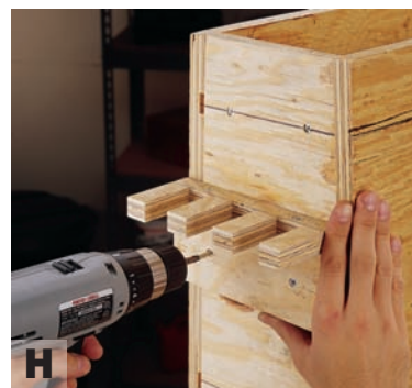
H Lay out the clamp holders and cut them to size. Notches 1 in. wide and 2 in. deep are a good size for holding standard pipe clamps. The bottom clamp holder can be made longer than the top, spanning across the end piece and the end divider.
